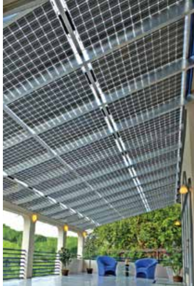
Patio Awning: Solar Living Design Lakewood, CO
